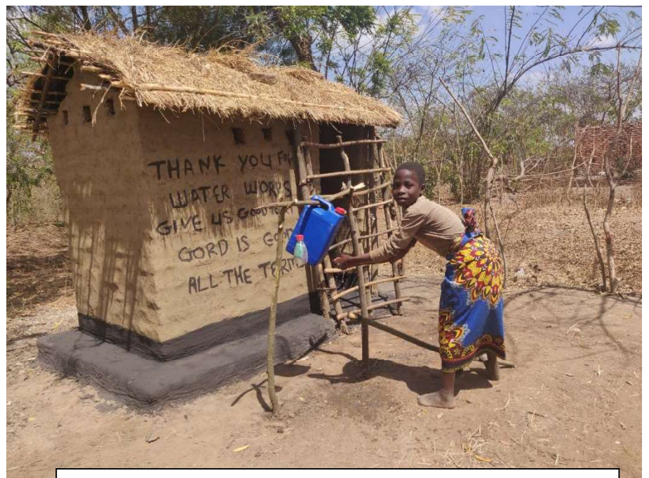
Girl washing hands with soap outside newly constructed latrine
